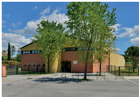
Gymnase Marcel Cau
