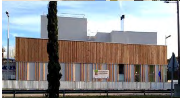
BHNS, chaufferie biomasse, Estelan
